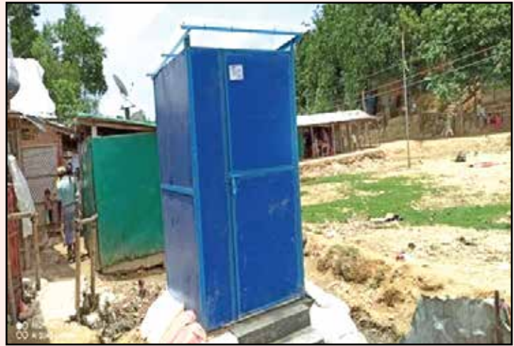
Bio-Fill latrine Installation in Camp
